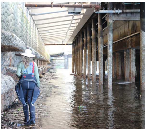
Figure 8.4a – In Seattle, salmon friendly seawalls have been built in the heart of their downtown waterfront. They are made up of glass sidewalks that allow light to dapple through to shallow rocky areas — to support salmon and their prey. Photo by: Bob Oxborrow
