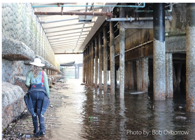
Figure 17 – In Seattle, salmon friendly seawalls have been built in the heart of their downtown waterfront. They are made up of glass sidewalks that allow light to dapple through to shallow rocky areas – to support salmon and their prey.
