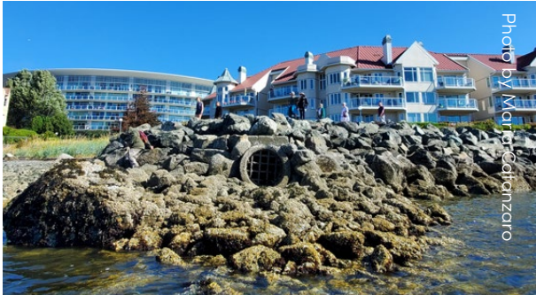
Stormwater outfall
